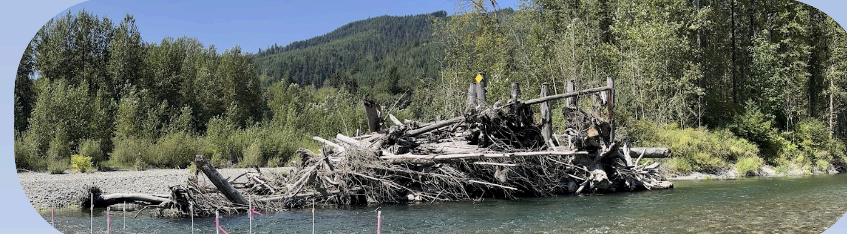
Engineered Log Jam (Site A2) on the South Fork Nooksack River, with piezometers in riverbed
